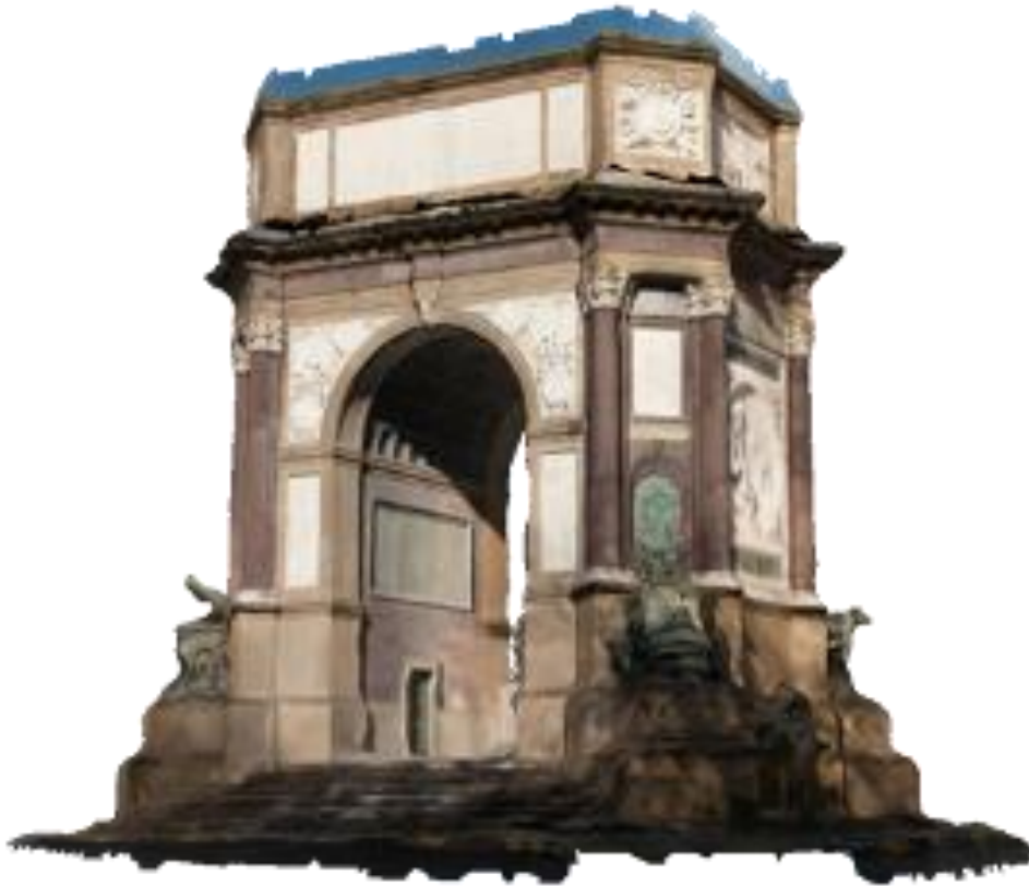
Figure 41: Result of applying the multi-texturing stage on the 3D mesh of Arco Valentino.
